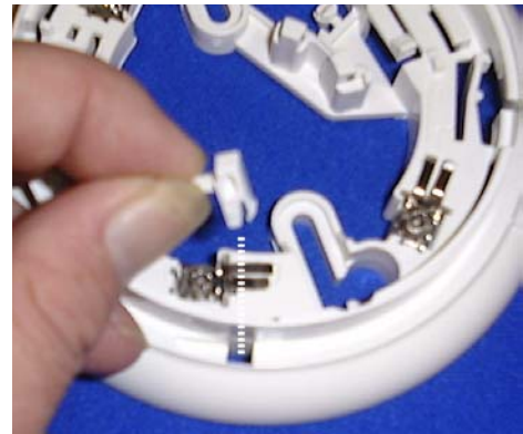
Fig. 9 Fitting Locking Device
